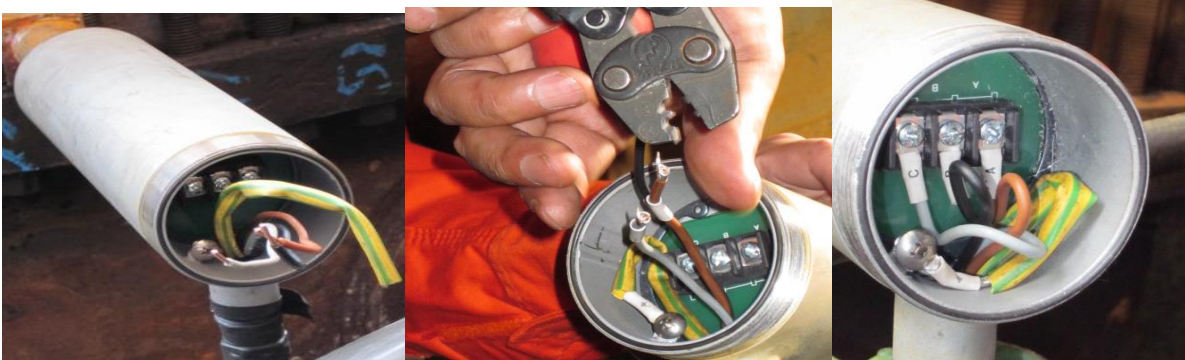
Figure 7: Transducer Wire Termination
