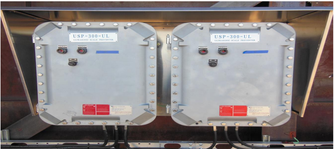
Figure 6: Typical installation: Generators with housing/shelter
