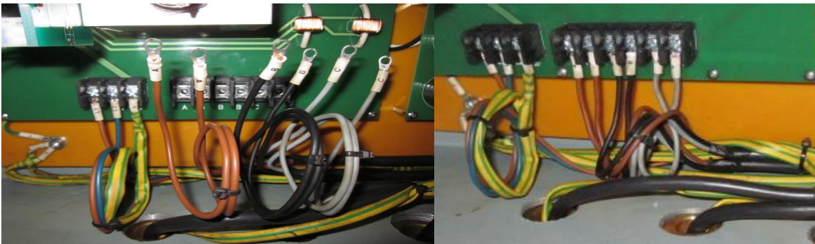
Figure 8: Generator Wire Termination
